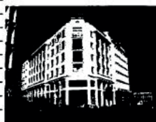
Building Abboud Abdel Razzak
